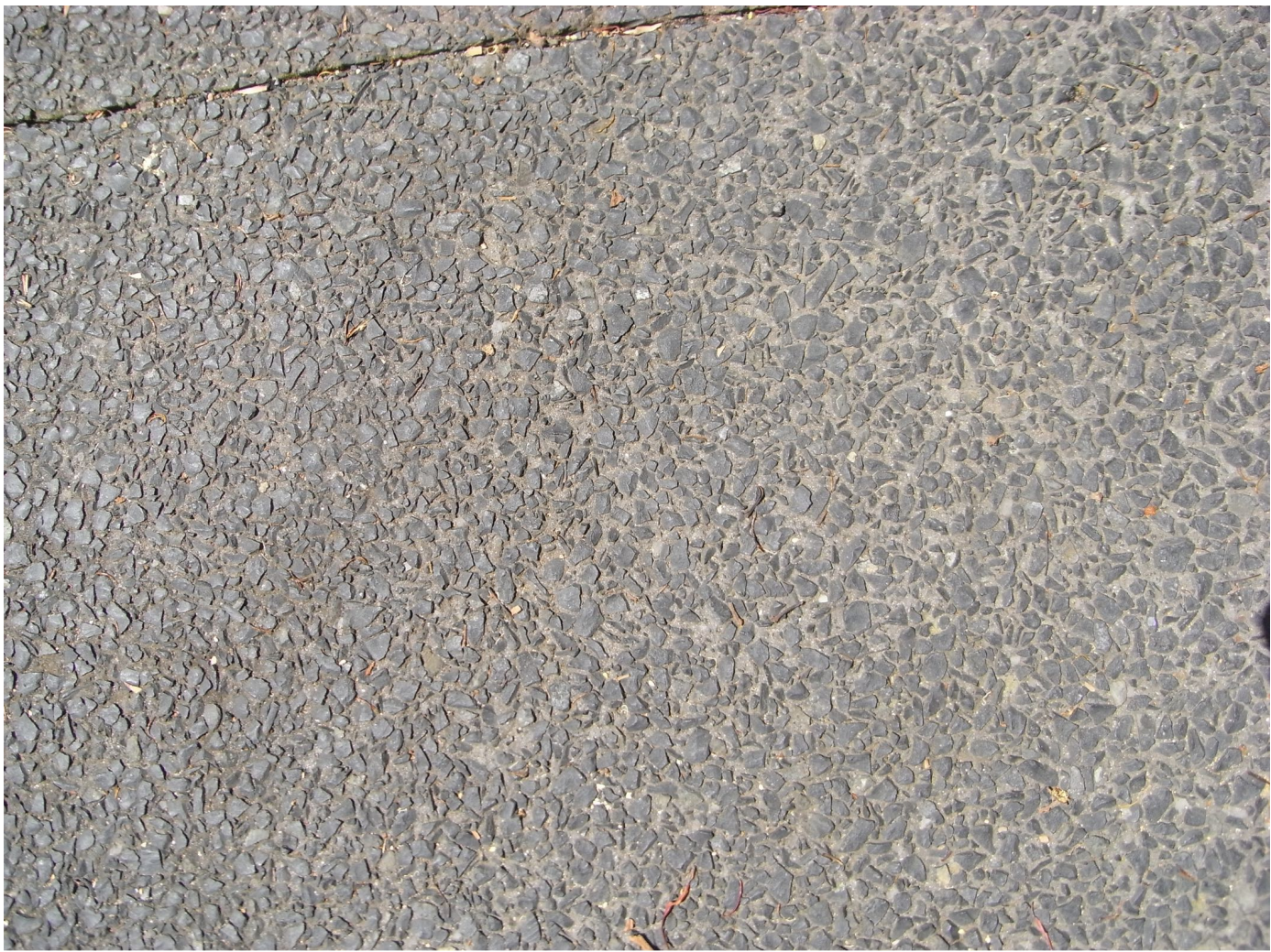
EXPOSED BLACK AGGREGATE FINISH WITH 300MM WIDE STENCILLED CONCRETE BORDER TO PERIMETER AND ACROSS DRIVEWAY AT NOMINAL 3000MM CENTRES (EXPANSION JOINTS) IN FULL DEPTH CHARCOAL COLOUR (AS AVAILABLE FROM BORAL).
